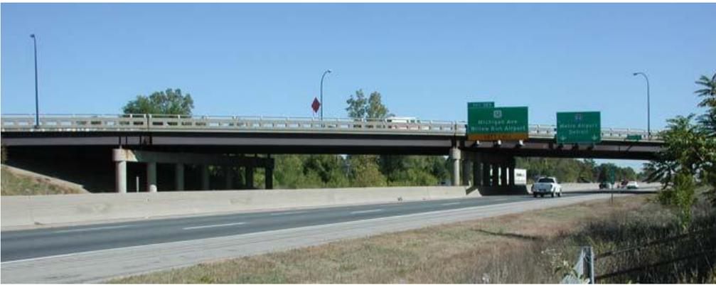
**Fig. 11.** Photograph of highway bridge in South-east Michigan where a SHCC link-slab was used in place of conventional expansion joint (Li, 2015)
