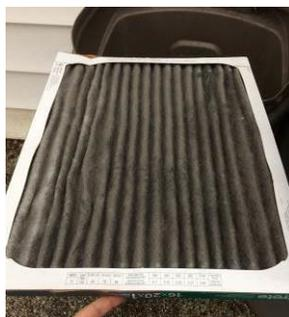
**Figure 2:** Dirty air filter to be replaced
