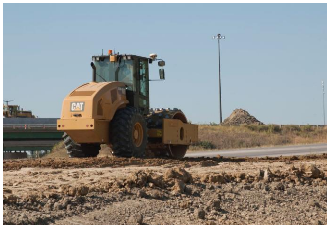
FIGURE 1 PADFOOT VIBRATORY SOIL COMPACTOR USING MDP TECHNOLOGY ON COHESIVE SOILS – IOWA USA
