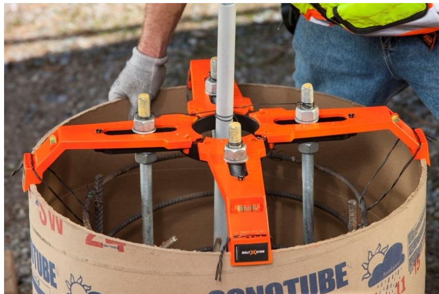
FIGURE 1 BOLT STAR INSTALLED ON FORMING TUBE
