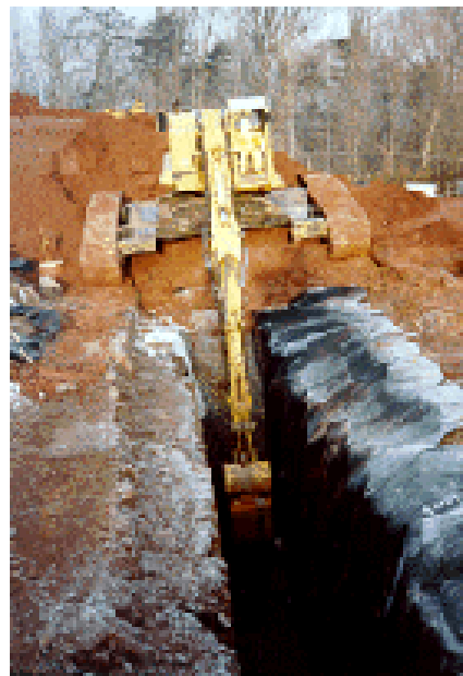
FIGURE 1 FUNNEL AND GATE SYSTEM EXCAVATION
