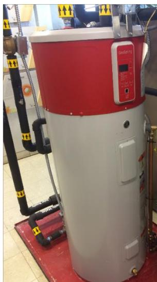
**Figure 3:** The residential air source heat pump has an integral storage tank.
