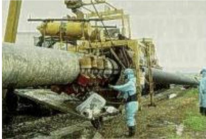
**FIGURE 2 HIGH PRESSURE WATER JET COATING REMOVAL EQUIPMENT AND CONTAINMENT SHROUD**
