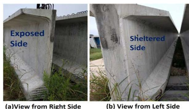
**Fig. 2.** Photos of a typical rejected girder showing (a) exposed side and (b) sheltered sides
