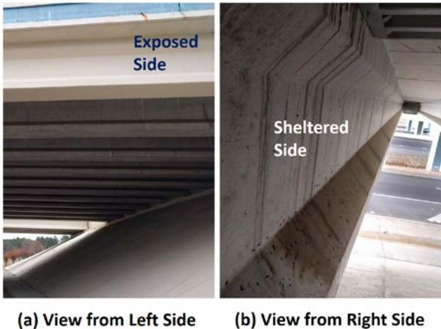
**Fig. 5.** In-service girder showing (a) exposed side and (b) sheltered side. Notice the exposed girder has been painted.
