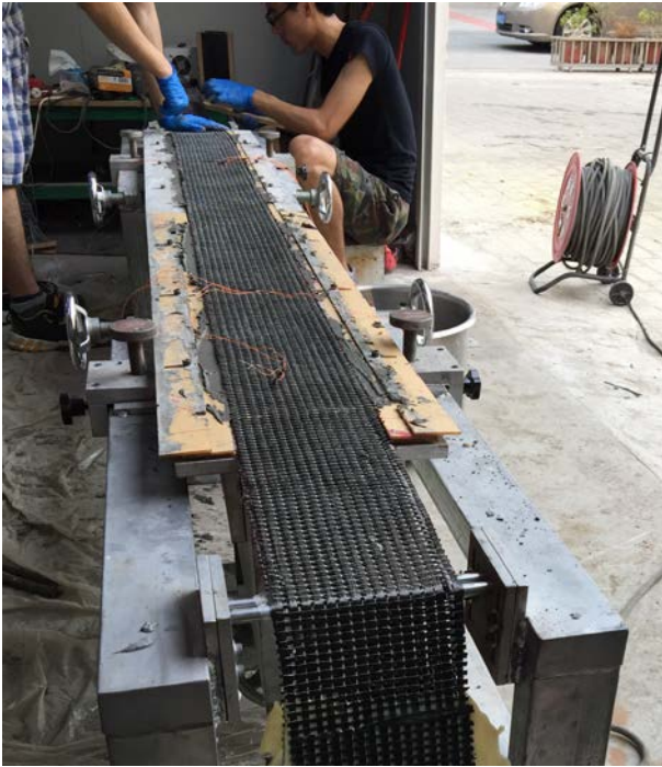
Fig.3. Installation of C-FRCM to the soffit of RC beams
