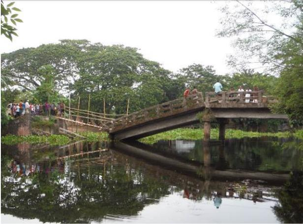
**Fig. 1.** Silna river road bridge collapse caused by erosion of river bed
