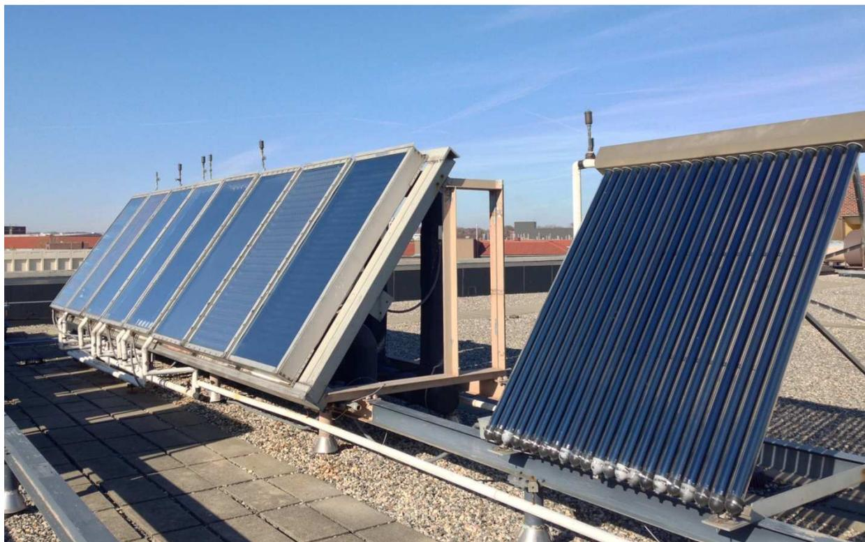
**Figure 2:** Solar thermal collectors on the roof of Knoy Hall
