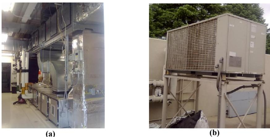
**Figure 9:** (a) Overview of air-handling unit (b) Overview of air-cooled liquid chiller
