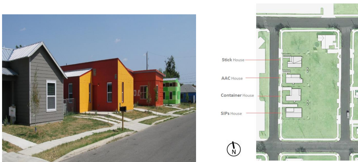
Figure 2: Four low income residential houses
