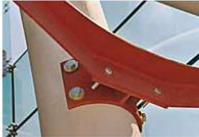
FIGURE 3 A FINISHED JOB WITH HOLLO-BOLT®
