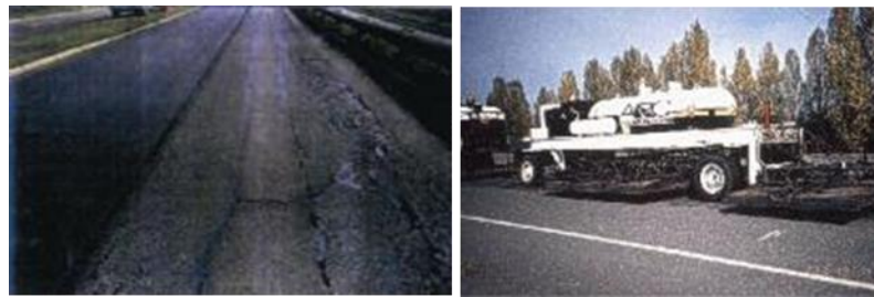
FIGURE 1 HOT IN PLACE ASPHALT RECYCLING (HIPAR)
