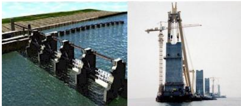
FIGURE 2 COMPLETED DAM IN OPERATION & VIEW OF HEAVY LIFT CRANE MOVING PRECAST ELEMENT
