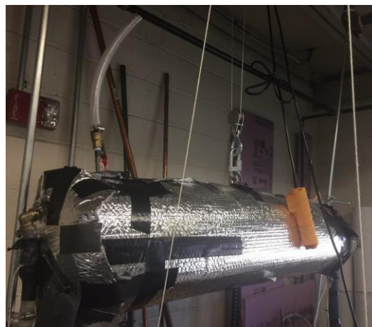
Figure 2(a) Storage tank for the indoor thermosiphon test facility.
