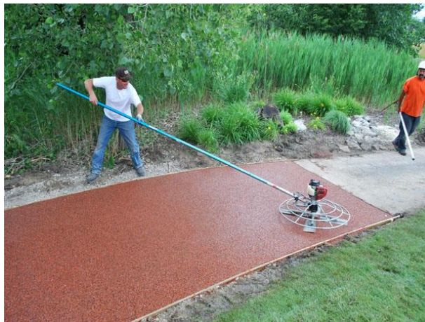
FIGURE 3 INSTALLATION OF FILTERPAVE SYSTEMS
