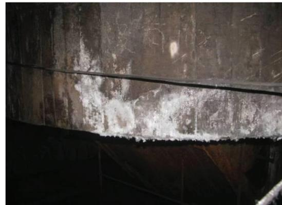
Figure 3. Funnel concrete surface with corrosive medium.
