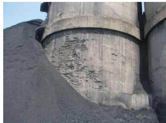
Figure 4. Damaged concrete wall of the bowl.
