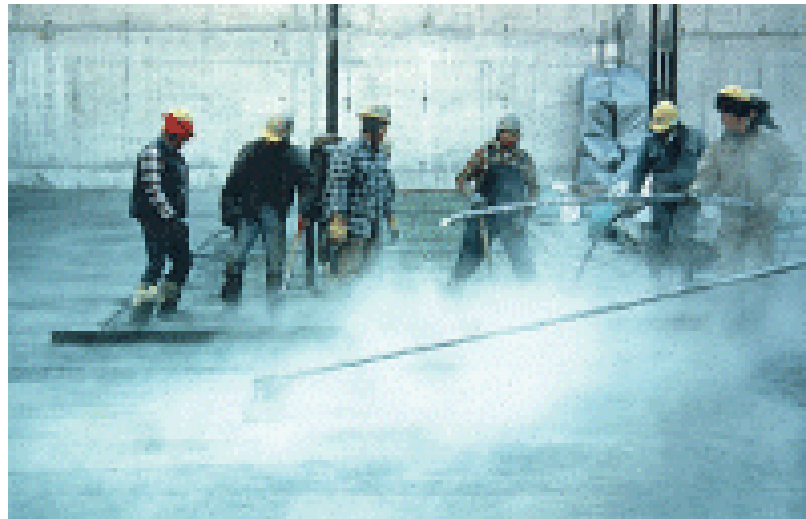
FIGURE 1 CONCRETE POURING IN THE LOW TEMPERATURE (COURTESY OF GRACE CONSTRUCTION PRODUCTS)
