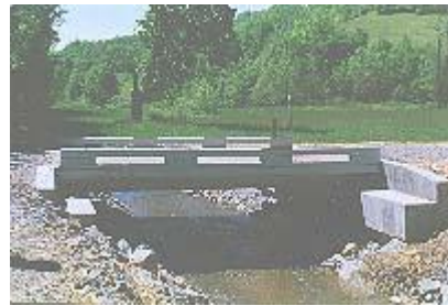
FIGURE 1 BEAMS ARE INSTALLED AT SITE
