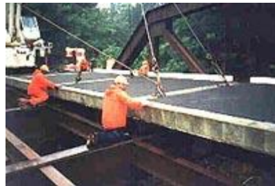
FIGURE 1 REHABILITATION OF A STEEL TRUSS BRIDGE
