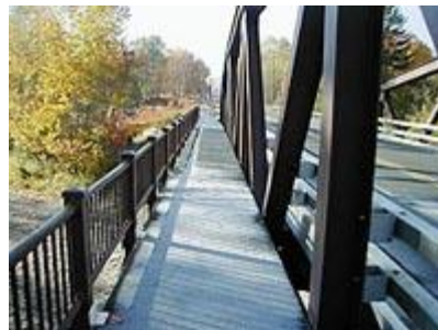
FIGURE 2 FRP DECK (A STEEL TRUSS BRIDGE)
