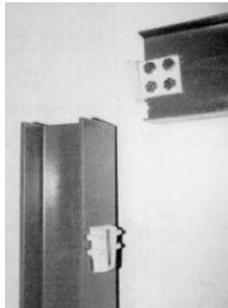
FIGURE 2 MORTISE ON COLUMN FLANGE AND TENON ON BEAM
