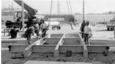
**FIGURE 3 BAY BEING ASSEMBLED ON GROUND**
