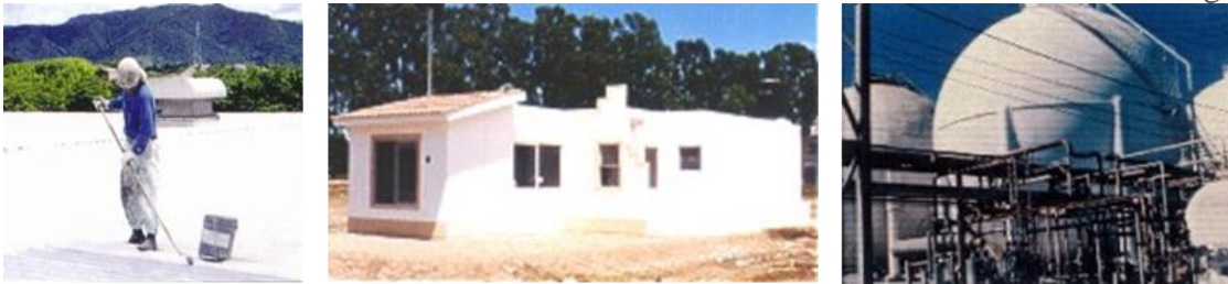
FIGURE 2 SUPER THERM APPLICATION (METAL ROOF/ CONCRETE WALLS/ SURFACE OF STORAGE TANKS)
