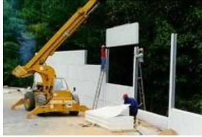
*Figure 4 Easy Panel Installation*
