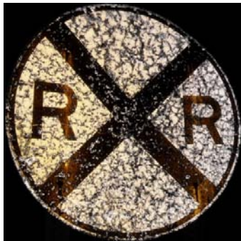
(c) Peeling of sheeting material.
