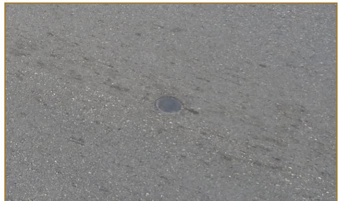
**Completed magnetometer installation.**
