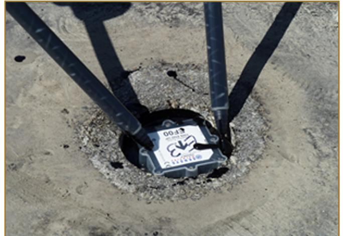
**Magnetometer installation: Filling core void with epoxy.**
