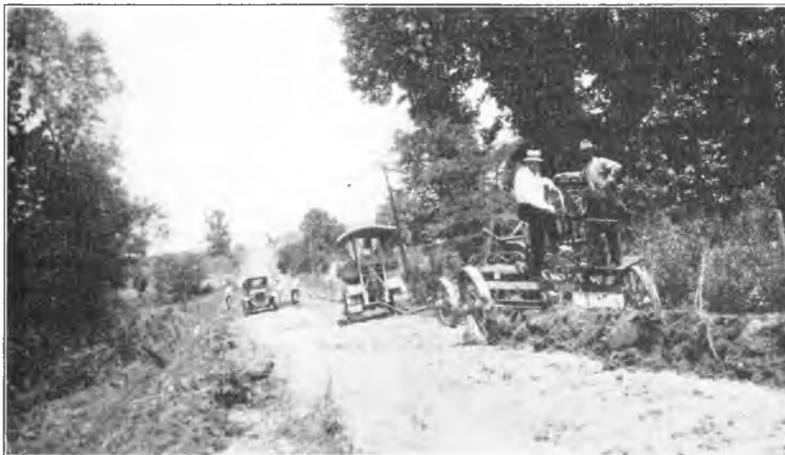
Fig. 2. Much work is needed in regrading and draining these narrow township earth roads.
