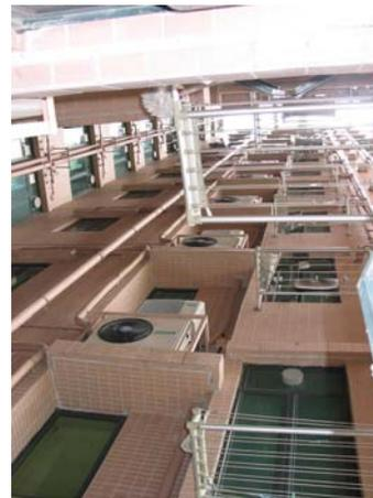
Figure 4 Installed outdoor units of split type air conditioners
