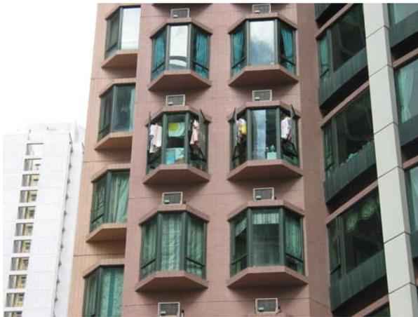
Figure 3 Installed window type air conditioners
