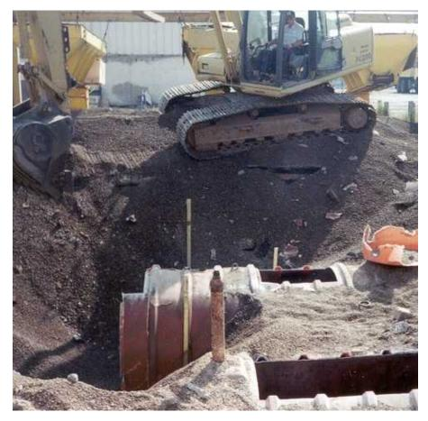
Figure 6. Excavator removing an underground storage tank
