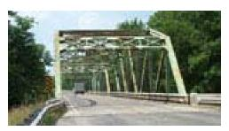
Figure 7. Many INDOT bridges have been painted with lead-based paint.
