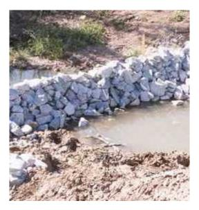
Figure 8. Soil erosion control implemented by INDOT
