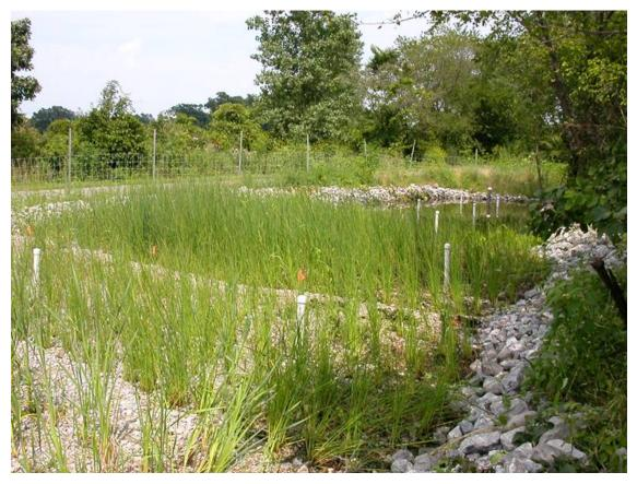
Figure 11. Interstate 65 site in late July 2003 showing the constructed wetlands.
