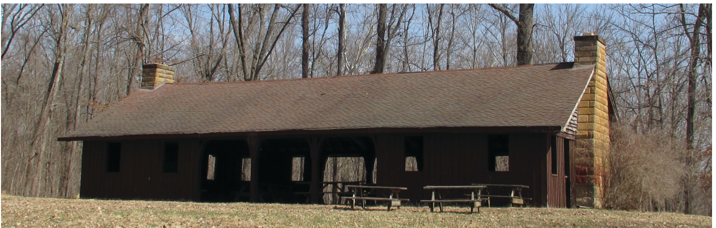
Figure 2. Wyandotte Woods State Park shelter house.
