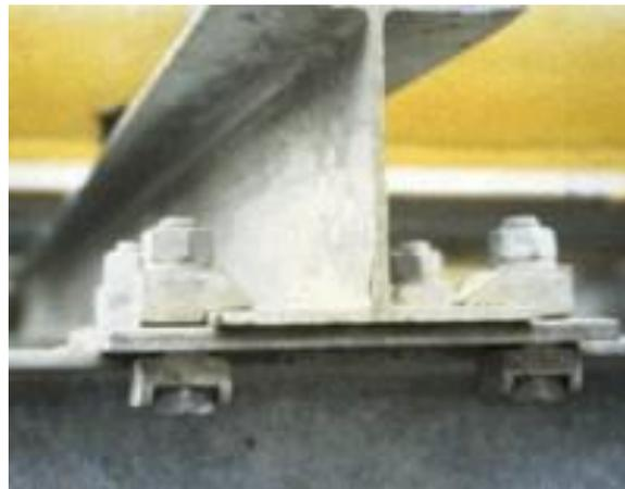
FIGURE 1 ADJUSTABLE STEELWORK CONNECTORS
