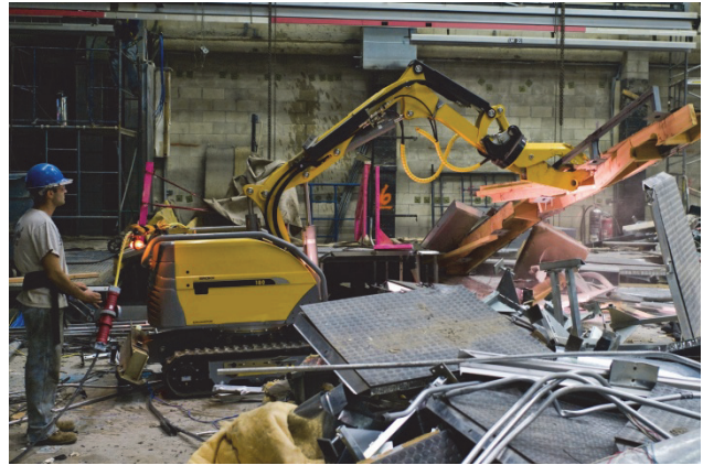
Figure 1. Remotely controlled demolition equipment
