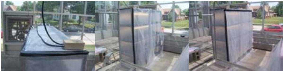
**Figure 2. Step-by-step construction of air-conditioned shelf: assembled plastic shelf bought a local home store; placement of a/c units; placement of lights; installation of reflective insulation; application of side plastic; sealing of plastic around a/c units; placement of timers; first layer of door plastic with slit down middle; and second flap of door plastic, held down with spring clamps.**
