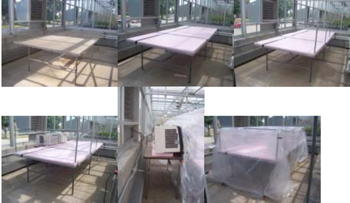
**Figure 4. Step-by-step construction of air-conditioned greenhouse bench: unmodified bench; placement of 2-inch foam board; placement of metal framing to create compartment; placement of a/c units near greenhouse fan; sealing of plastic around a/c units; two layers of clear plastic draped over frame, weighted down with spring clamps.**
